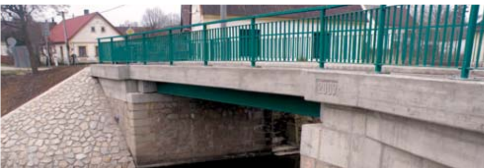
4 Bridge over Mlýnský potok (creek) in the village Lasenice
