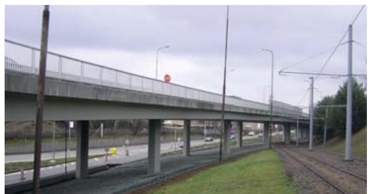
6 Scaffold bridge on I/52 at the central cemetery in Brno
