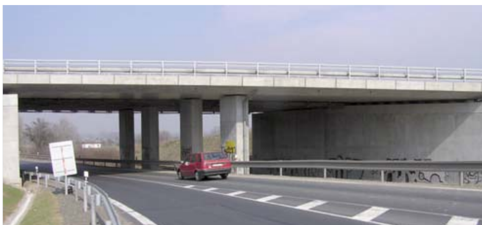
2 Bridge on the D1 highway in Kroměříž
