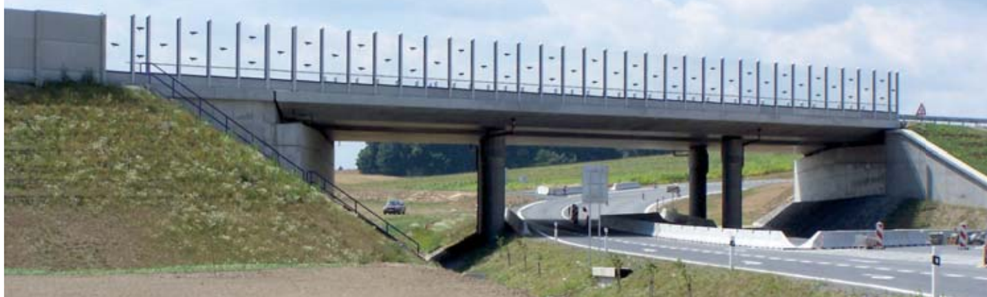
1 Bridge over the road I/47 in Běloutín
