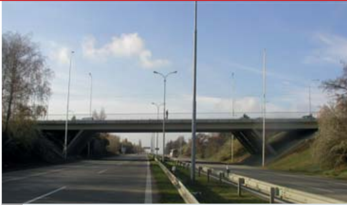
1 Bridge Holzova over street Ostravská, Brno
