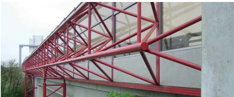
2 Noise barrier wall near the bridge D1-181 right near Velké Meziříčí
