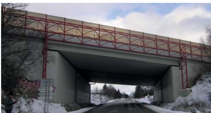
5 The bridge No. D1-181 near Velké Meziříčí
