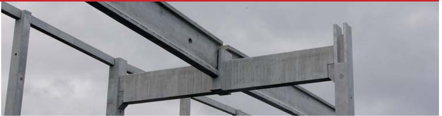
1 Cromodora Wheels - roof trusses for the factory buildings
