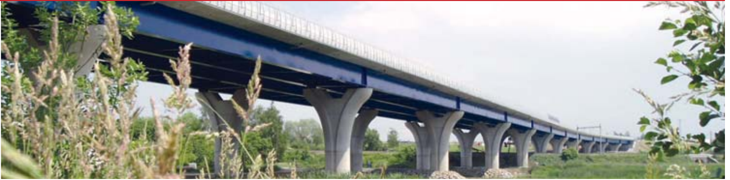
1 Scaffold bridge on the R48 on by-pass road Běloutín
