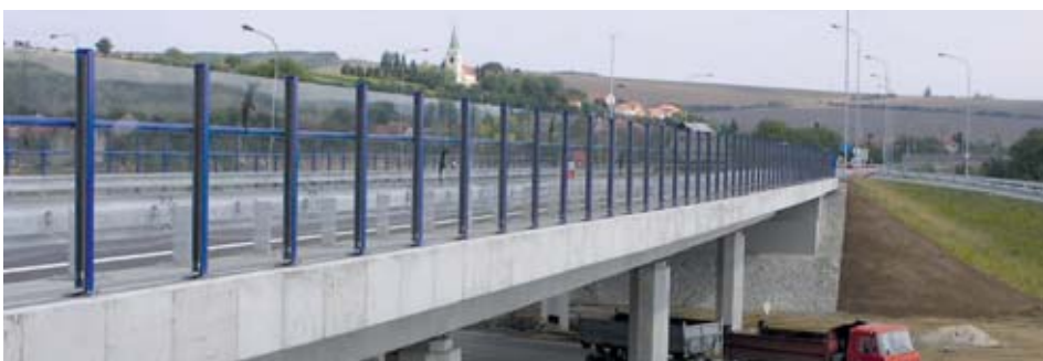
4 Noise barrier wall on the road viaduct in Uherské Hradiště
