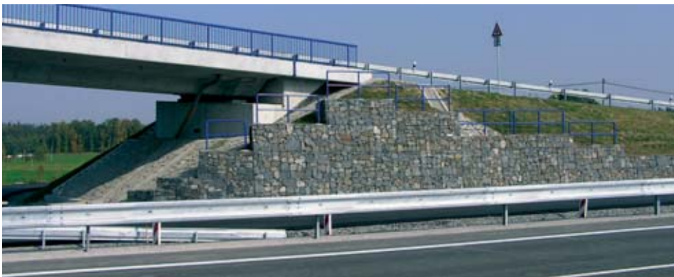
2 Gabion retaining wall on the road I/48 Dobrá - Tošanovice
