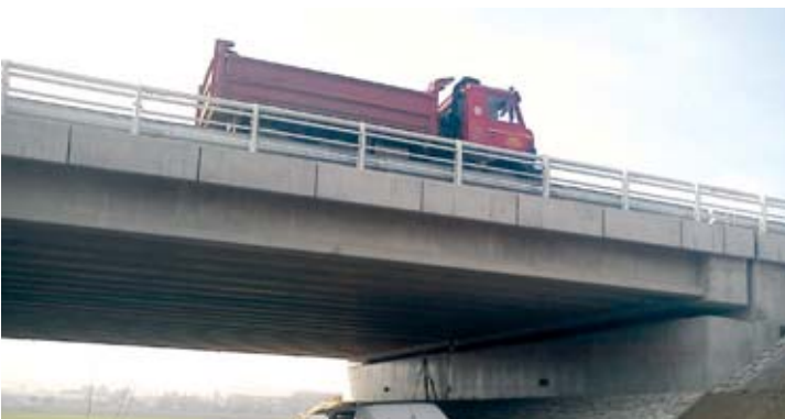
4 Bridge over the road I/47 at Lipník nad Bečvou
