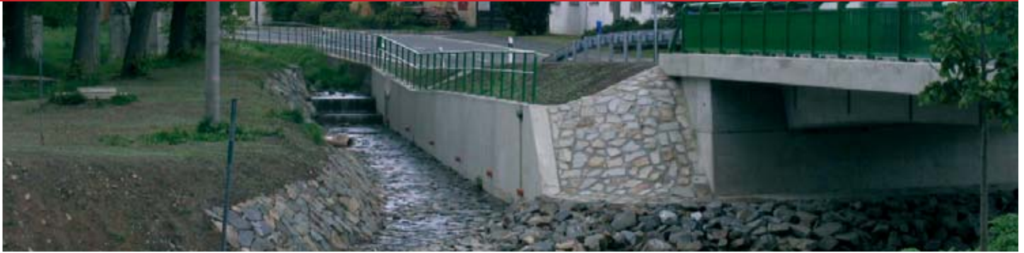
1 Retaining wall in the village Písečné
