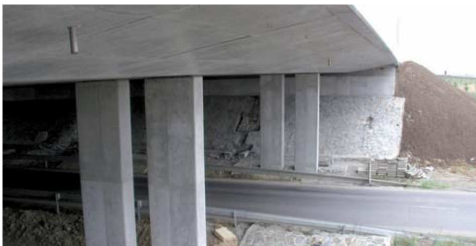
3 Bridge over the local road and biocorridor
