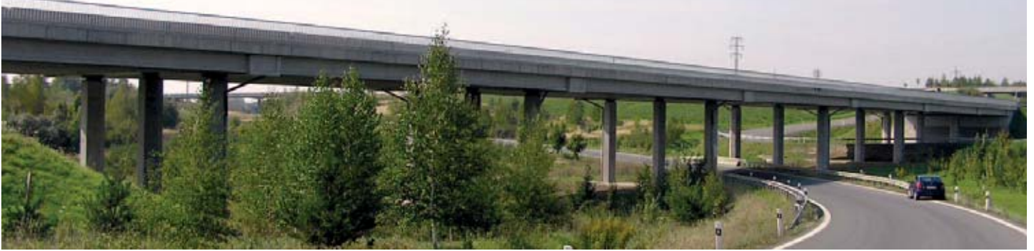
1 Scaffold bridge across the landfill on the R35 at the Lipník nad Bečvou
