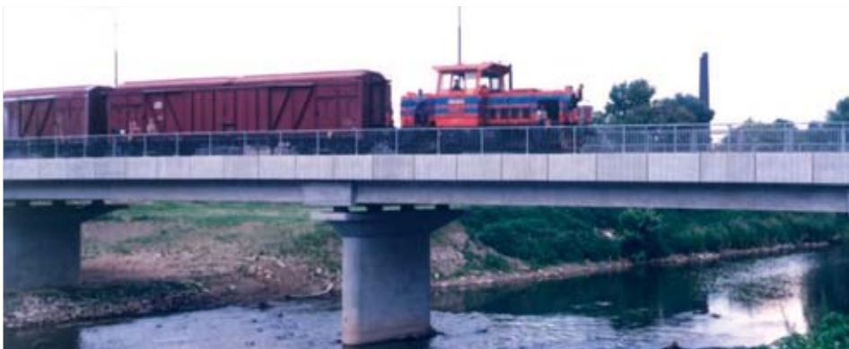
2 Railway bridge for siding of Precheza Corporation in Přerov over Bečva River
