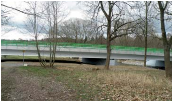
3 The bridge over the Volyňka River near the village Nišovice
