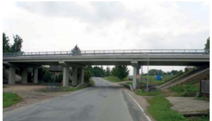
4 The bridge on the road I/38 near the village Habry
