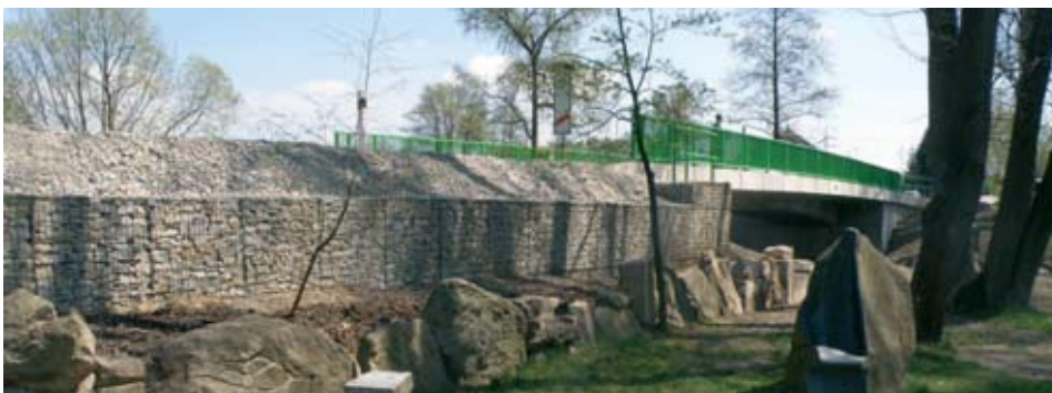
3 Gabion retaining wall at the bridge in Dolní Skrýchov
