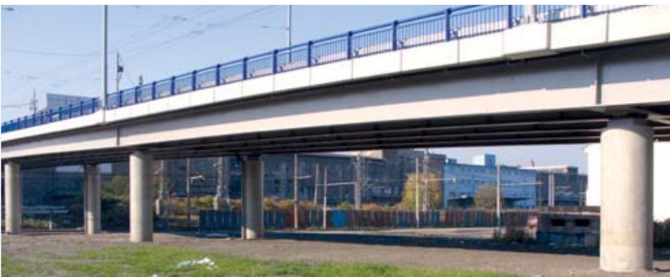
2 North Bridge in the street Českobratrská in Ostrava
